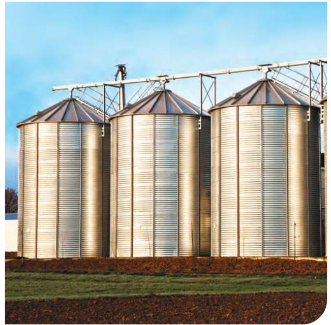
Figure 24–8: The gas formed during fermentation of crops stored in a silo can kill a person within minutes if inhaled.
